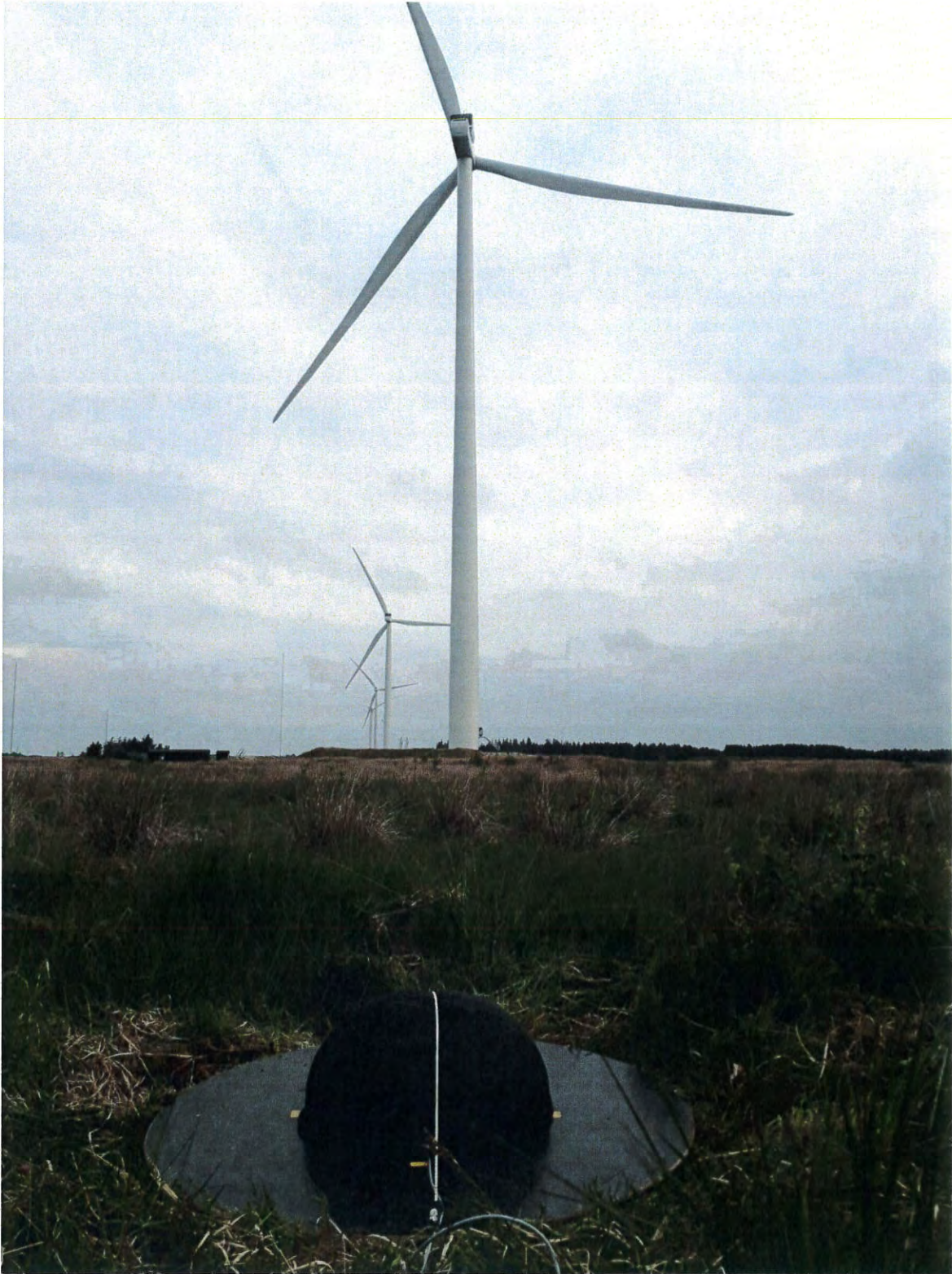
Photo 1: Measured turbine of the type Vestas V150-4.2 MW 50 Hz
