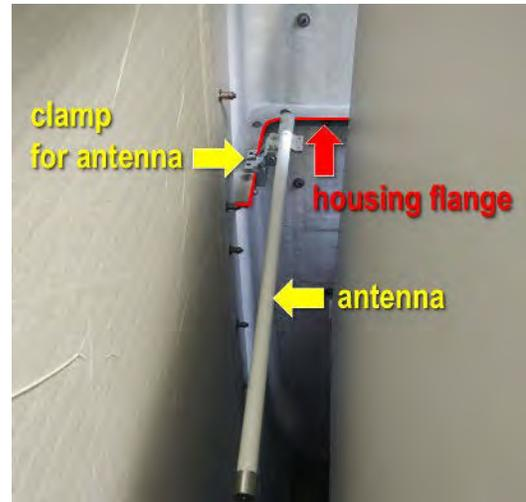
On request, the receiving antennas can also be mounted on nearly every fixture inside and outside the nacelle or on ground near the turbine. Other example is shown below for outside installation:
