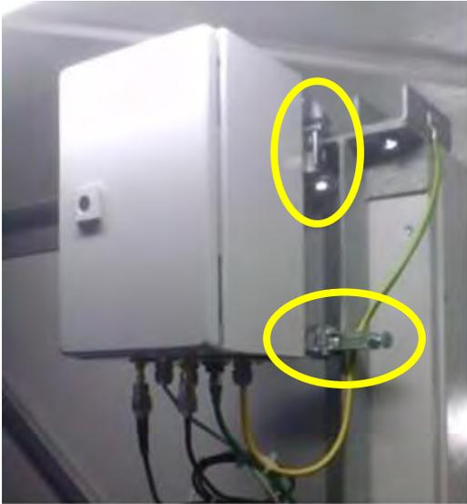
Option B (on request only): mounting brackets for fixation to IPS profile (on request): Rittal brackets No. 2508.100 can be supplied pre-mounted to the corners of the device.
